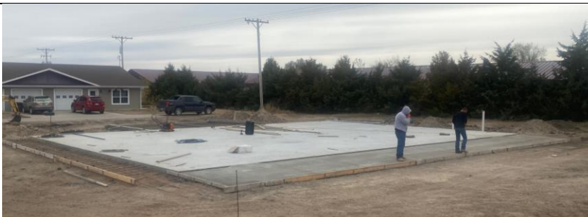
Foundation's daycare duplex under construction.
